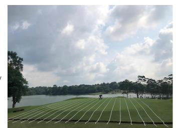
Potter said: "The initial trials I saw were showing how this drainage element could pull water from Point A to Point B on surfaces with no falling grade, and they even showed me how it could pull water uphill as long as the end of the drainage element was lower than the starting point.
