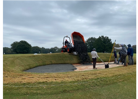
Capillary Bunkers' liner system was chosen at Carolina Golf Club 'to seal off the clay'. Picture by Matthew Wharton.
